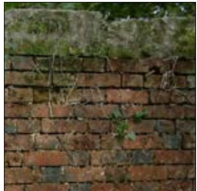
Shanklin Manor: the east garden wall and 'summerhouse' with a close up view of the stone coping and brickwork facing into the garden
