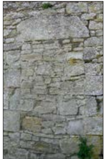
Barton: the terraced walled garden and stone lintel over a blocked entrance
