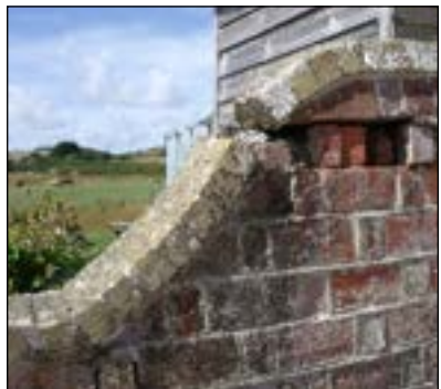
Castlehurst: brickwork detail
