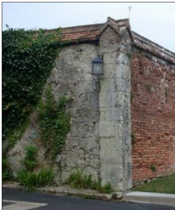
Appuldurcombe: the southwestern outside corner of the former walled kitchen garden
