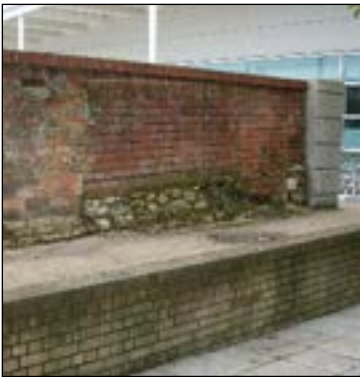
The Lodge: the two sides of the former southern kitchen garden wall with modern brick coping and extended plinth base
