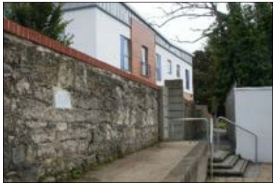
The Lodge: the two sides of the former southern kitchen garden wall with modern brick coping and extended plinth base
