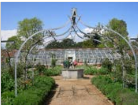
Osborne: the restored 1854 lean-to greenhouses in 2014
