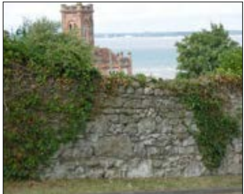
Egypt House: external view of the eastern stone boundary wall
