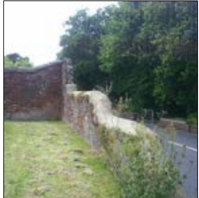
Appley Tower: parts of the former kitchen garden walls
