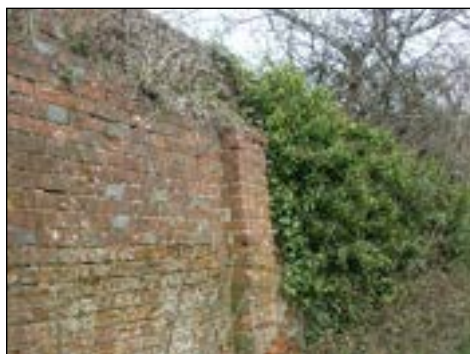
Bembridge Lodge: the southeastern boundary wall on High Street
