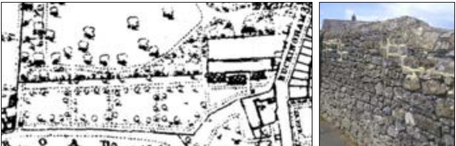
Buckingham Villa: the walled kitchen garden on the the 1864 OS and a section of the kitchen garden southern boundary wall on Spencer Road
