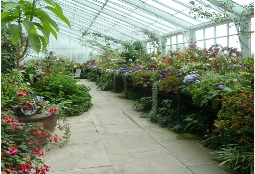
Restored glasshouse Wallington, Northumbria. Photo by Kate Harwood.
